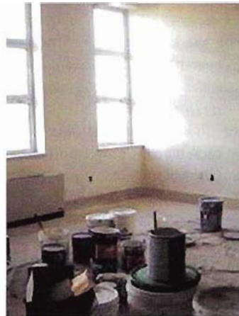
Before: Dining room is a construction mess!
